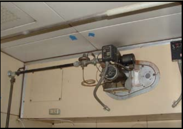
Original and still functional Gas-o-matic furnace surrounded by labeled interior panels. —Marlene Terreros-Oronao, May 3, 2006
