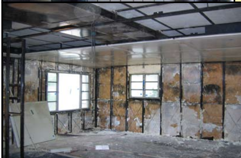
View of second bedroom looking northwest, with exposed wall framing, ceiling panels, plenum, and fiberboard insulating panels above. The plenum is the black rectangular box extending below the insulating panels and above the ceiling panels. —Charles Craig, May 18, 2006
