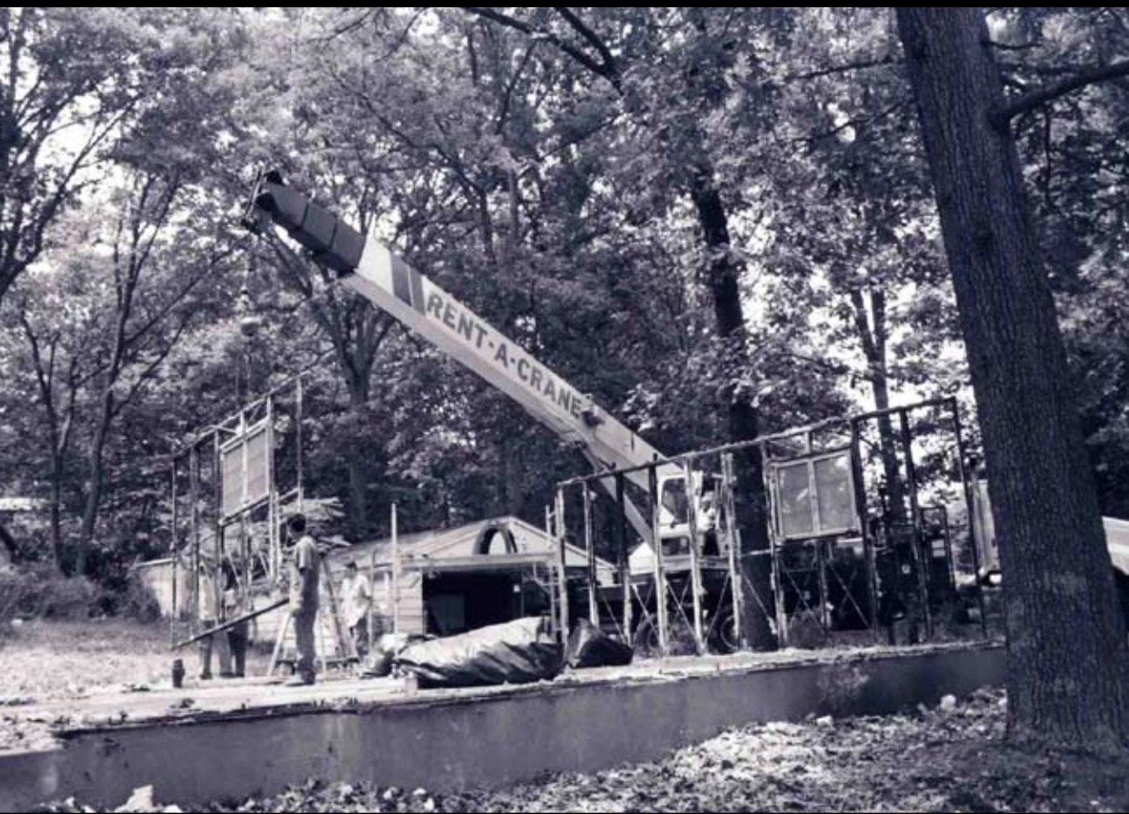
Removal of the first section of the right (north) wall in the rear bedroom. —Victor Muniec, June 8, 2006
