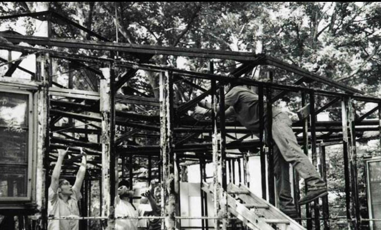
The whole crew adjusts the fallen roof trusses that collapsed upon removal of the first truss. —Cynthia Liccese-Torres, June 8, 2006
