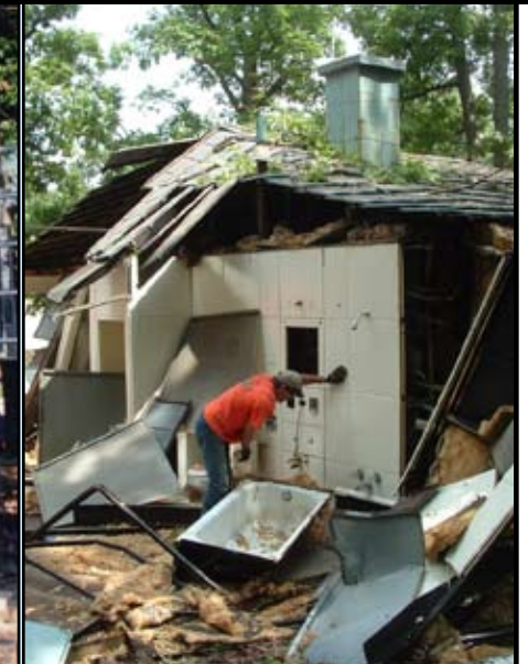
Freeing the bathtub, once the excavator partially demolished the bathroom. —Cynthia Liccese-Torres, August 10, 2005
