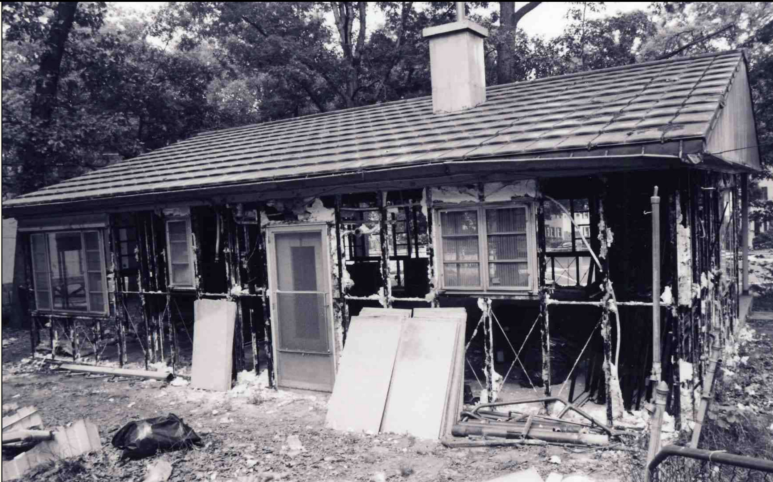
View of rear (west) elevation with all exterior panels and insulation removed. —Victor E. Muniec, May 2006
