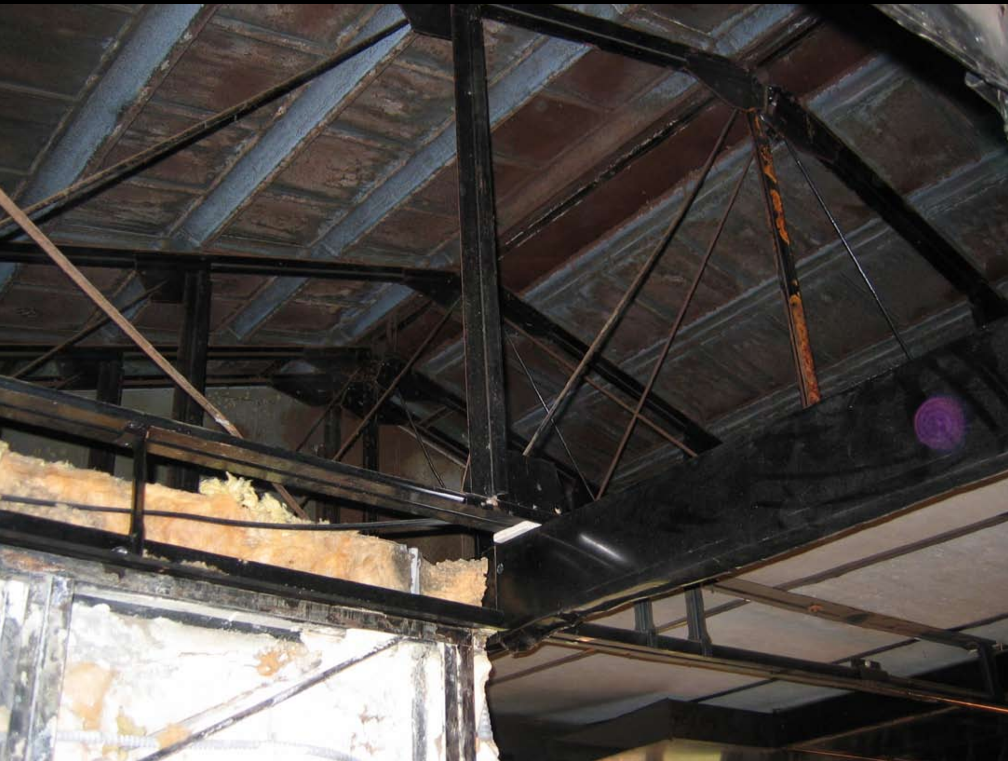
Detail of exposed roof trussing and underside of roof panels. —Charles Craig, May 18, 2006
