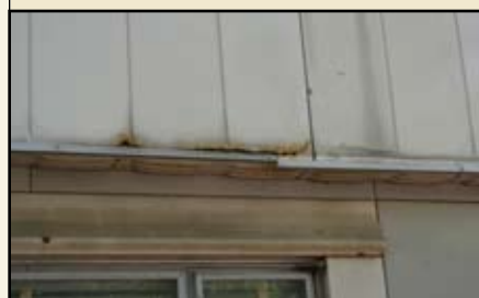
Detail of rusting at base of vertical panels along the gable ends. —Todd Zeiger, May 3, 2006
