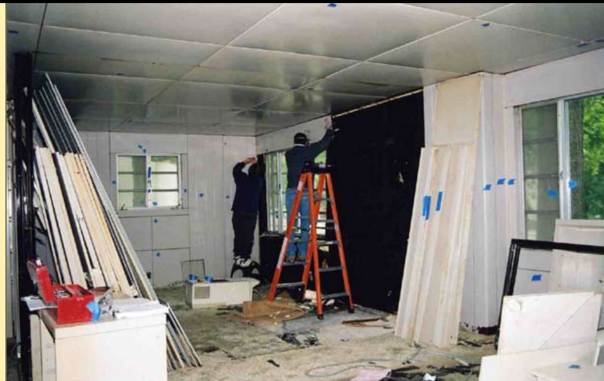
Interior wall panels being removed along the front wall of the master bedroom. —Victor E. Muniec, May 5, 2006
