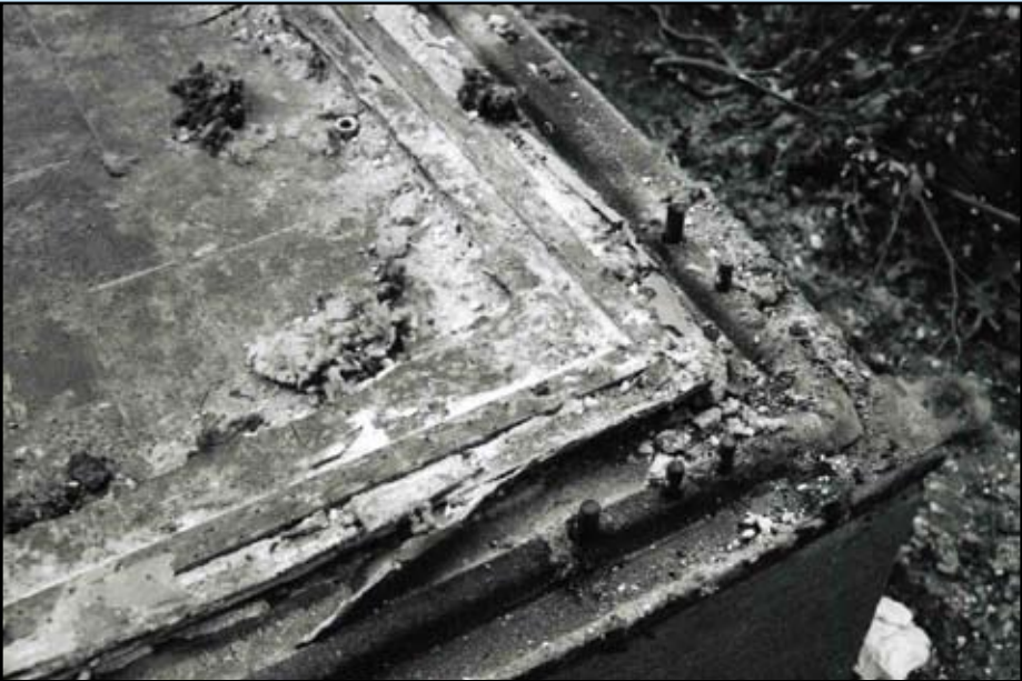
Detail of the metal tracking attached to the perimeter of the foundation where the wall sections were anchored. This tracking could not be salvaged from the Krowne Lustron site. —Cynthia Liccese-Torres, June 8, 2006
