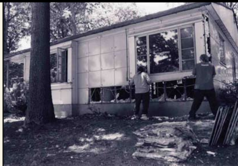
Removal of the first exterior panels on the front elevation; note the pile of fiberglass insulation from the panels stacked on the front lawn. —Victor E. Muniec, May 2006
