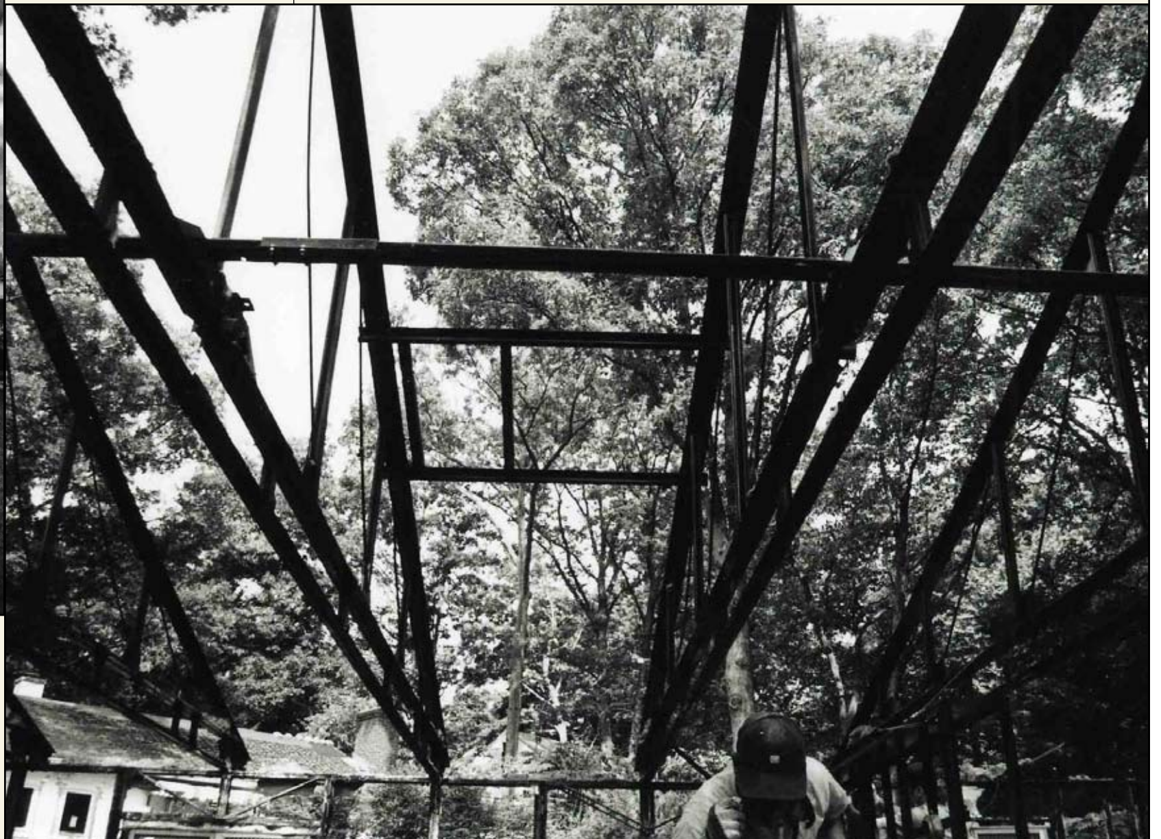
Detail of roof trusses looking up through the roof; note the rectangular opening in the middle for the chimney flue. —Cynthia Liccese-Torres, June 8, 2006
