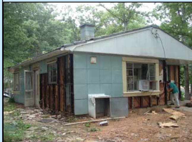
Rear and left side elevations, showing salvaged panels and exposed wall framing. —Cynthia Liccese-Torres, August 10, 2005
