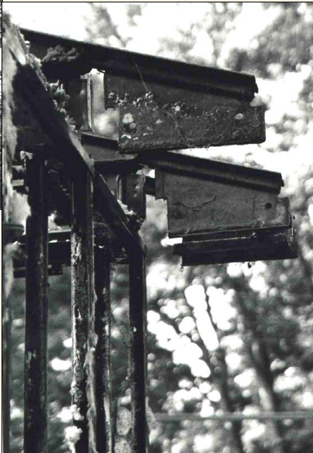
Detail of ends of roof trusses at southwest corner of house. —Cynthia Liccese-Torres, June 6, 2006
