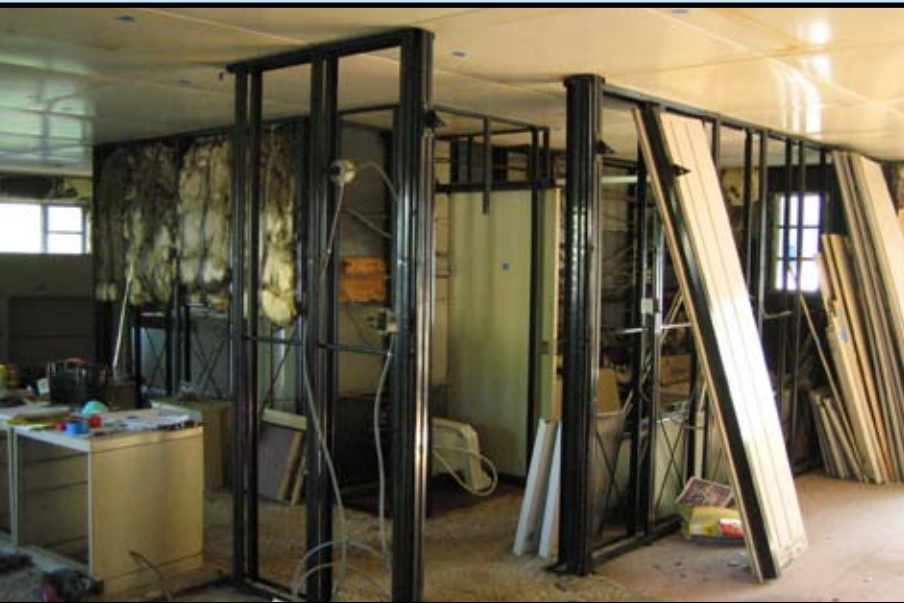
Interior paneling is partially removed, showing the wall sections comprising the bathroom, hallway, and utility room. —Tom Dickinson, May 2006
